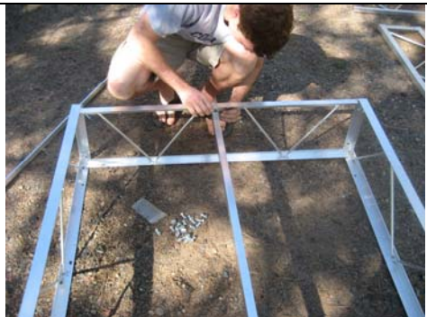
Install End Rail on last frame
