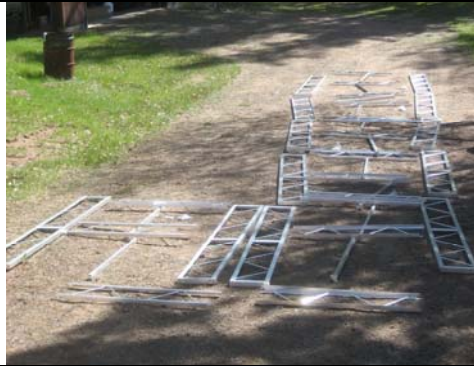
Lay out frames
