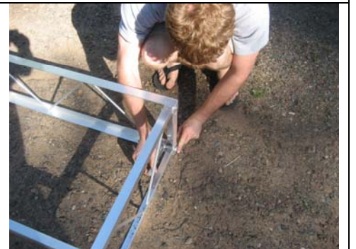
Tighten all frame bolts
