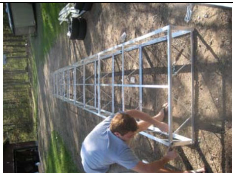
Continue tightening bolts
