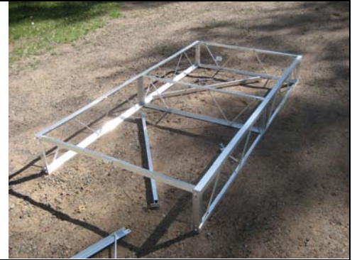
Loosely assemble 1 st frame
