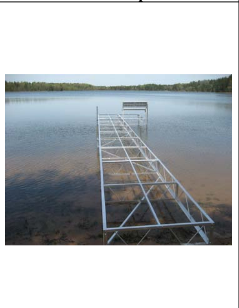
Completed frame in water
