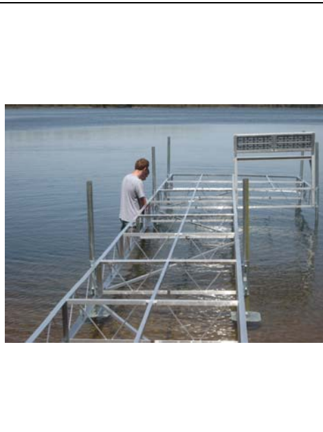
Level dock frame in water
